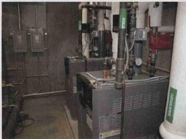
High efficiency LAARS boilers.
