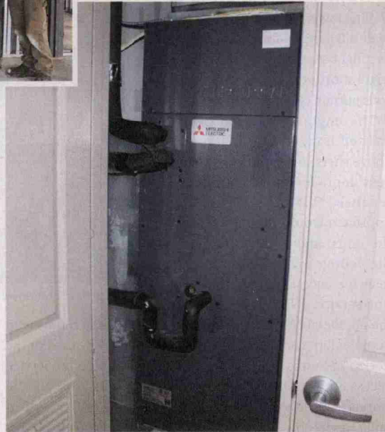
One of the Mitsubishi Electric City-Multi heating and cooling systems in place.
